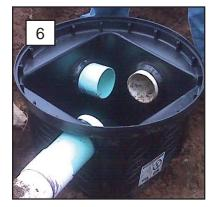
You are now ready to insert the correct size pipe by pushing it through the flexible watertight D-Box seal.
