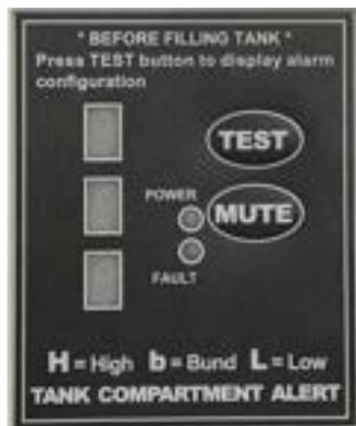
Alarm configuration is displayed when the **TEST** button is pressed & held.
