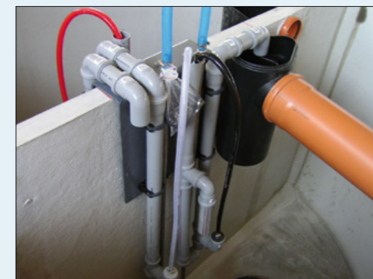
Image shows System pack for retrofitting > 28 inhabitants)
