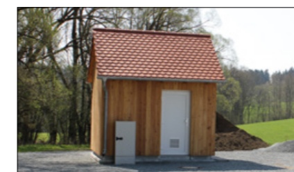
Example: Installation in a machine house
